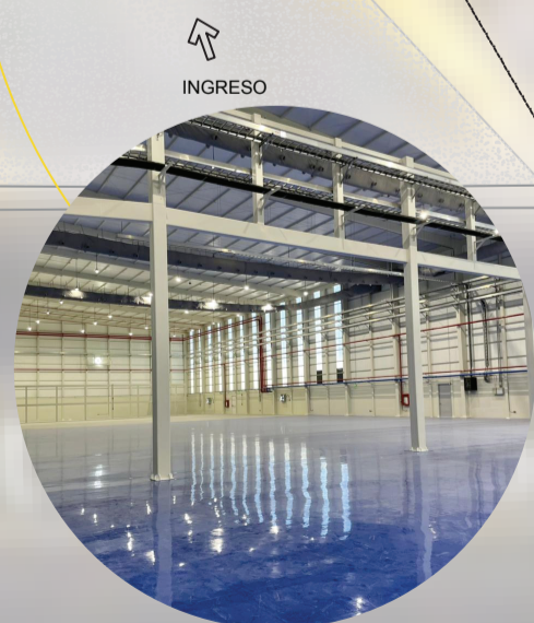
FADESA PLANT ILLUMINATION
